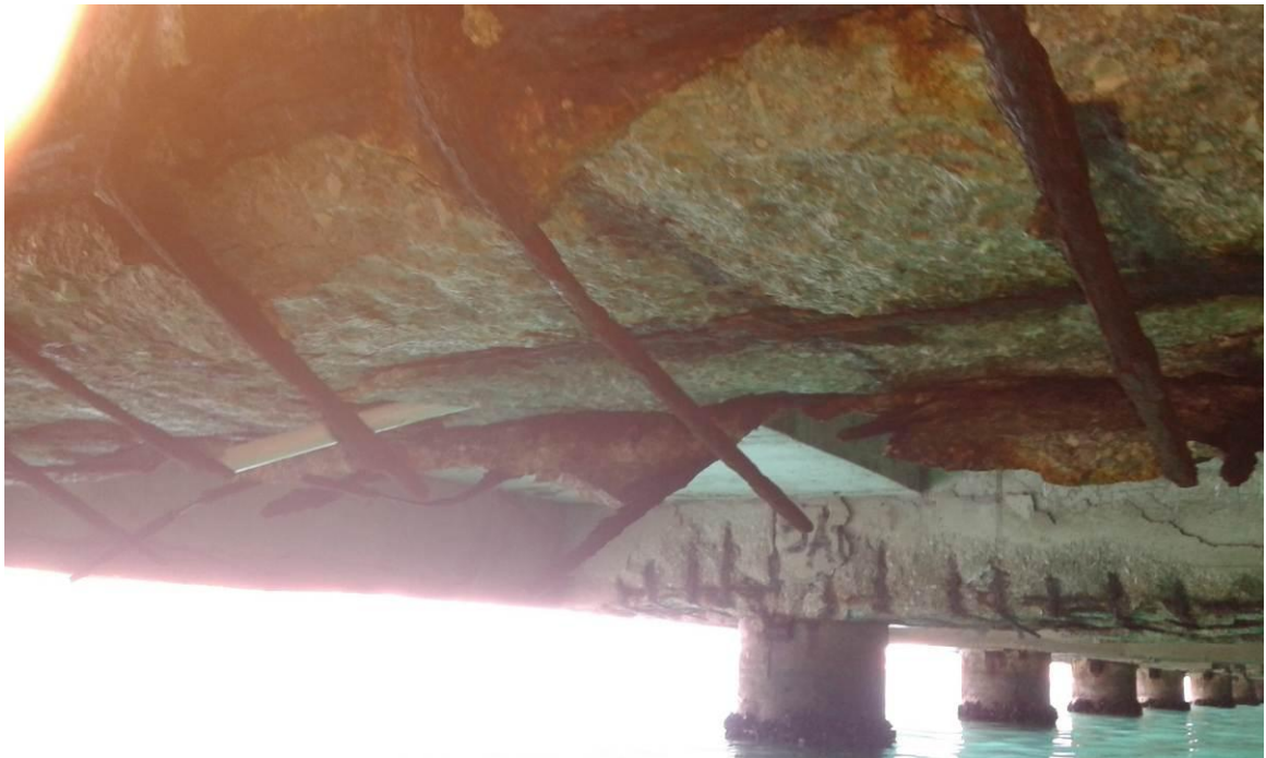
Picture 5.b) Damage TYPE 1 – longitudinal and transverse reinforcement of transverse beams has completely corroded and prolapsed from the original position. Diameter of the reinforcement is significantly reduced
