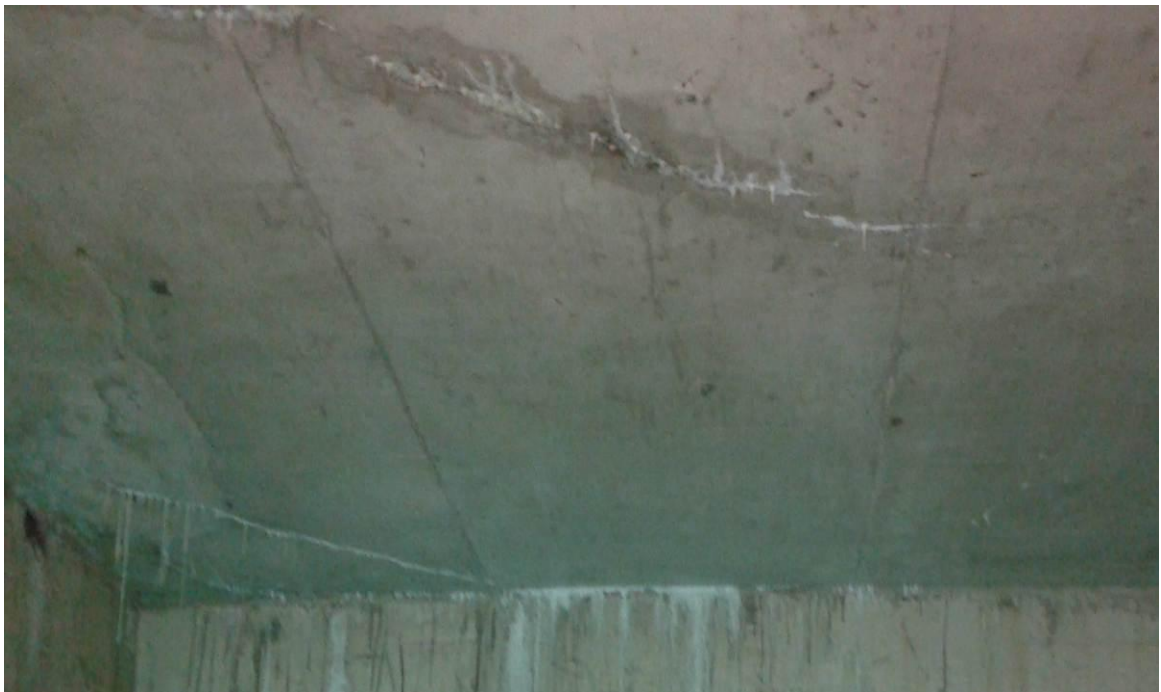
Picture 10. Damage TYPE 2 – Damage of the slab in the form of concrete falling off in thin layers and surface damage due to carbonization
