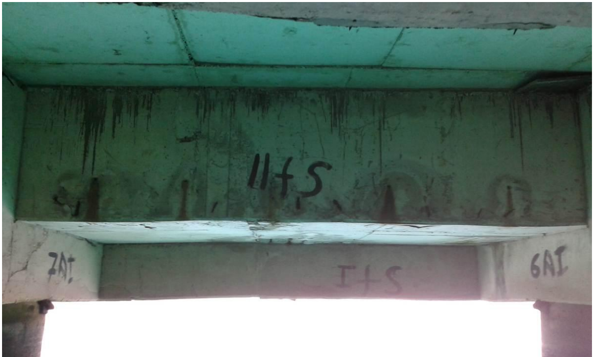
Picture 9. Damage TYPE 2 – Damage of lower slab of boxed girder and longitudinal beams in the form of concrete husking, peeling and falling off in thin layers
