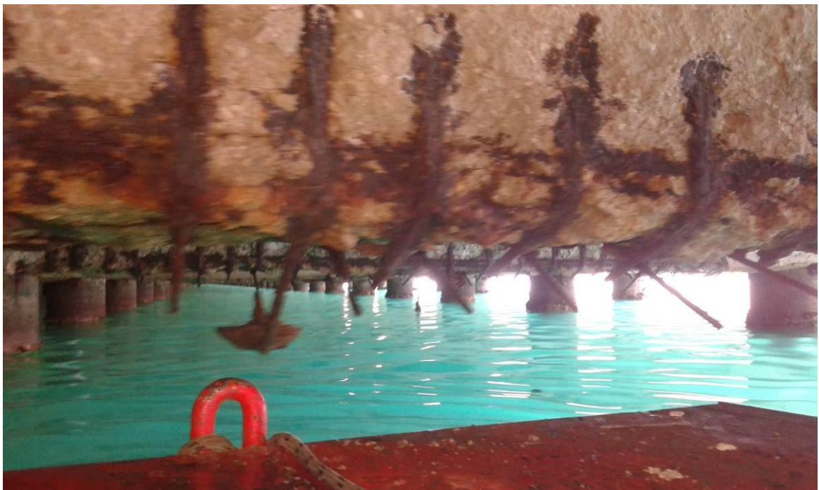
Picture 5.c) Damage TYPE 1 – longitudinal and transverse reinforcement of transversal beams has completely corroded and prolapsed from the original position. Diameter of the reinforcement is significantly reduced
