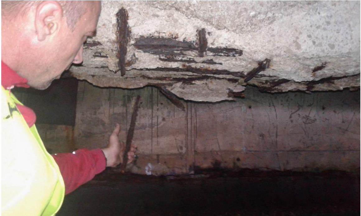
Picture 5.d) Damage TYPE 1 – Detail of breaking by hand of part of transversal reinforcement from transverse beam
