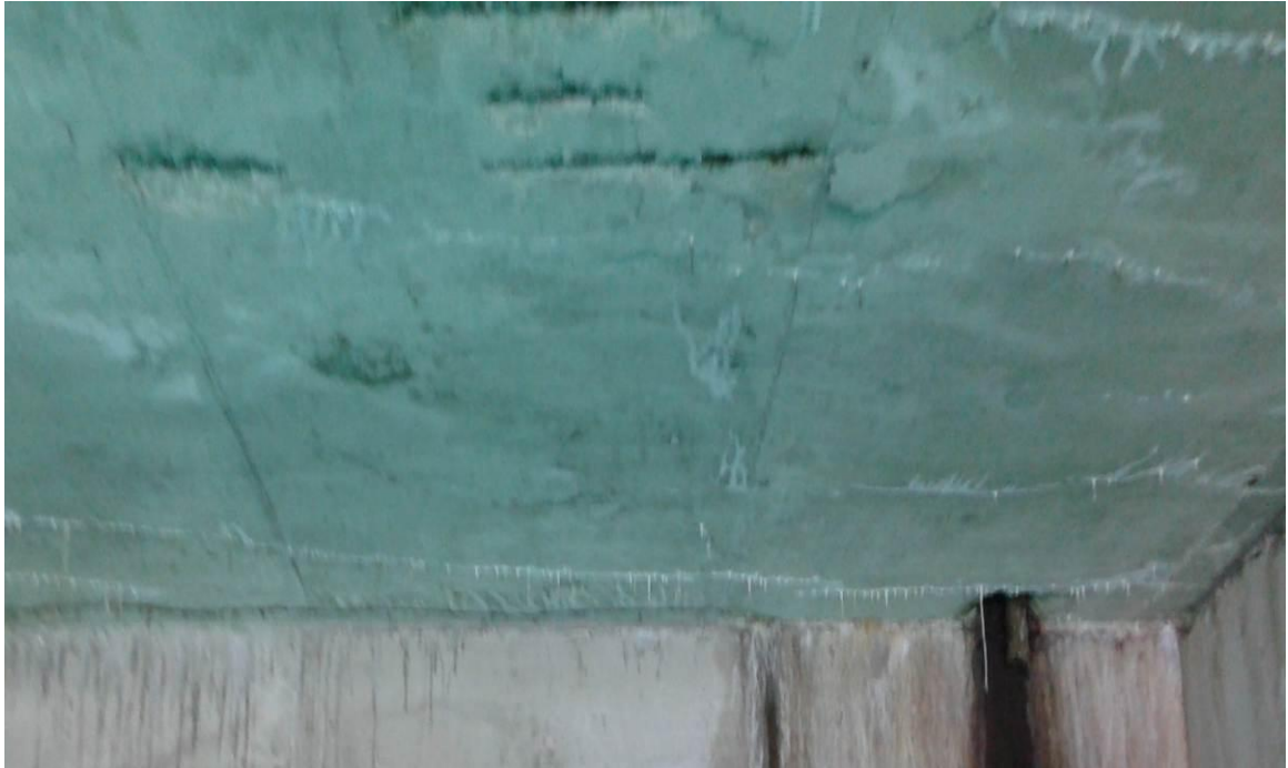
Picture 7. Damage TYPE 1 – RC slab damaged in the form of concrete falling off up to visible reinforcement and peeling off concrete in layers
