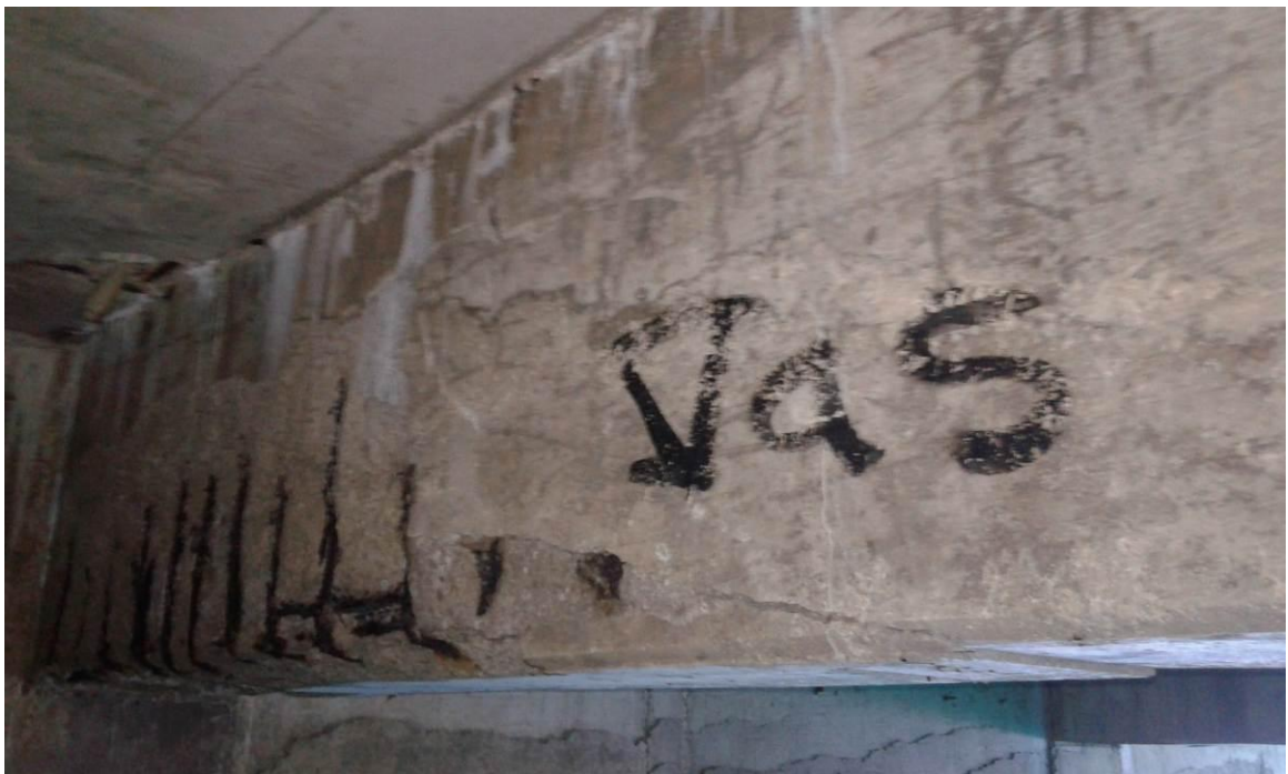
Picture 6. Damage TYPE 1 –Damage of longitudinal beam in the form of block falling off, up to visible transversal reinforcement and one row of longitudinal reinforcement
